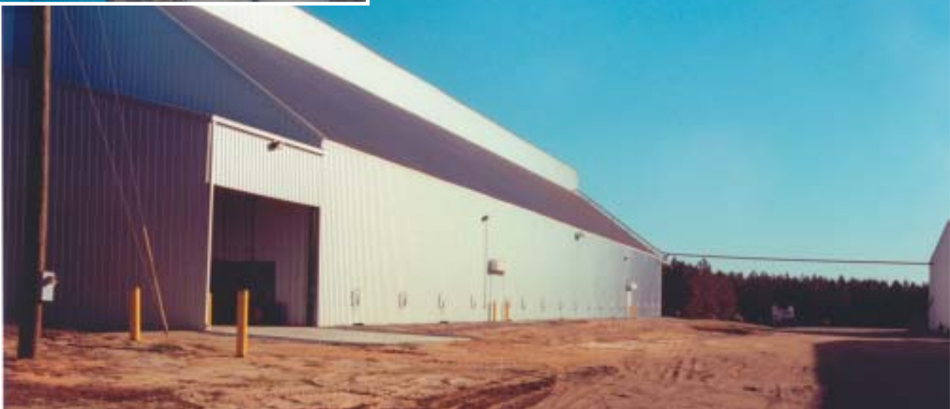
The 28,800 square foot warehouse can store up to 35,000 tons of peanuts and cottonseed.
